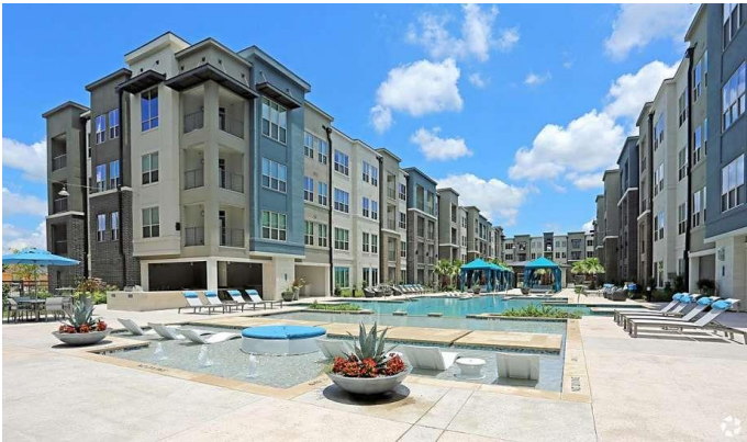
Multi Dwelling Units
